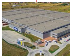
Dacia Warehouse, Pitesti
