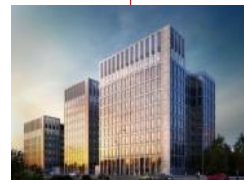
A4 Business Park, Katowice
