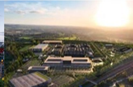
AiOnX data centre development fund
