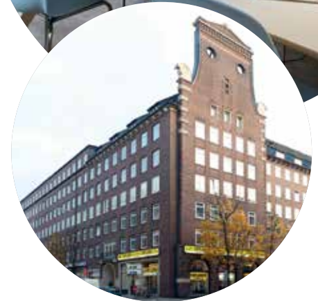
The refurbished Bartholomayhaus in Hamburg's historic Kontorhausviertel
