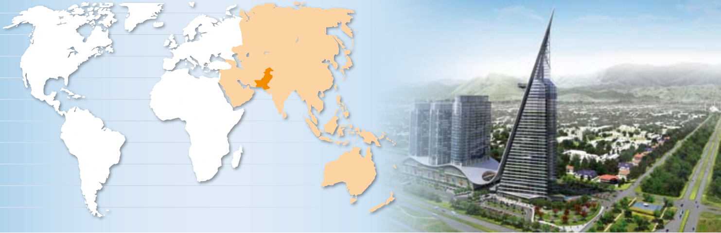
The Centaurus is a mixed-use development project currently under construction in Islamabad, Pakistan.
