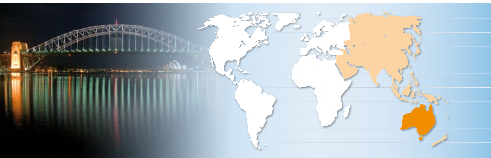
Sydney harbour bridge.
